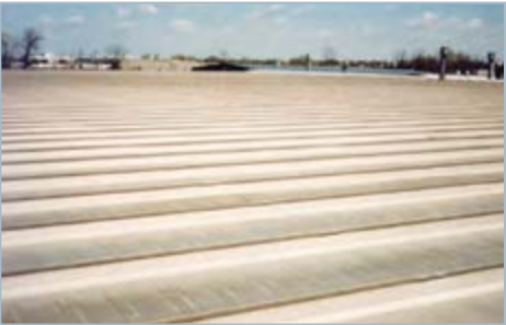
G/L roof 20 years at light industrial area
